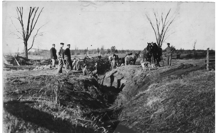
Workmen digging the drainage ditch from Peterson Lake to the Embarrass River are shown in a photo from the 1930s.
